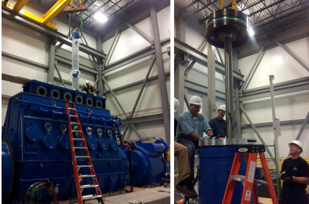
Figure 2: Left: Test-fit of a SustainX HP cylinder on top of the lower-half of a MAN engine (crankshaft). A PMG can be seen to the right of the crankshaft. Right: Installation of a LP piston into a LP cylinder.
