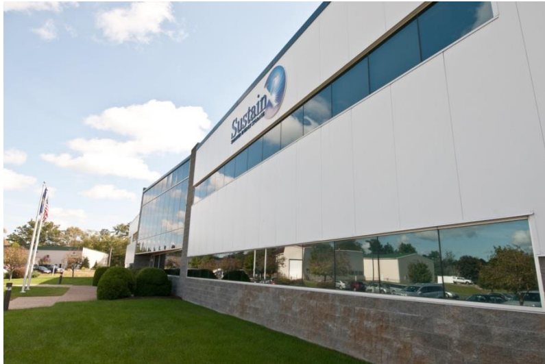
Figure 1: SustainX facility in Seabrook, New Hampshire
